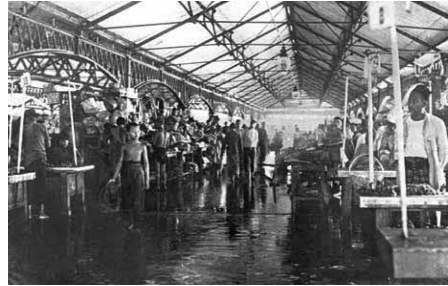
The interior of Telok Ayer Market showing the cast iron by MacFarlane and Company in Glasgow, 1910s. The market (more popularly known today as Lau Pa Sat or "Old Market" in Hokkien) opened in 1894. Courtesy of National Archives of Singapore.
